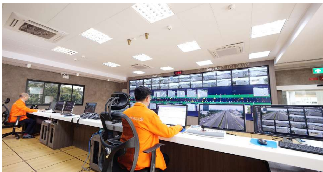
Operation Control Center: OCC
